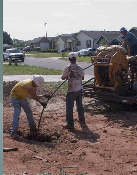
Pipe Loop Insertion
